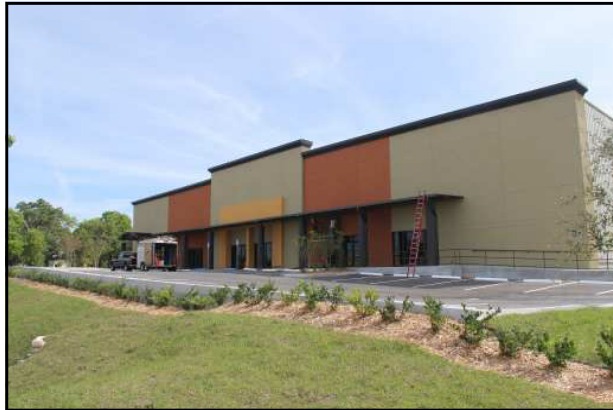
Rear Building—under construction
